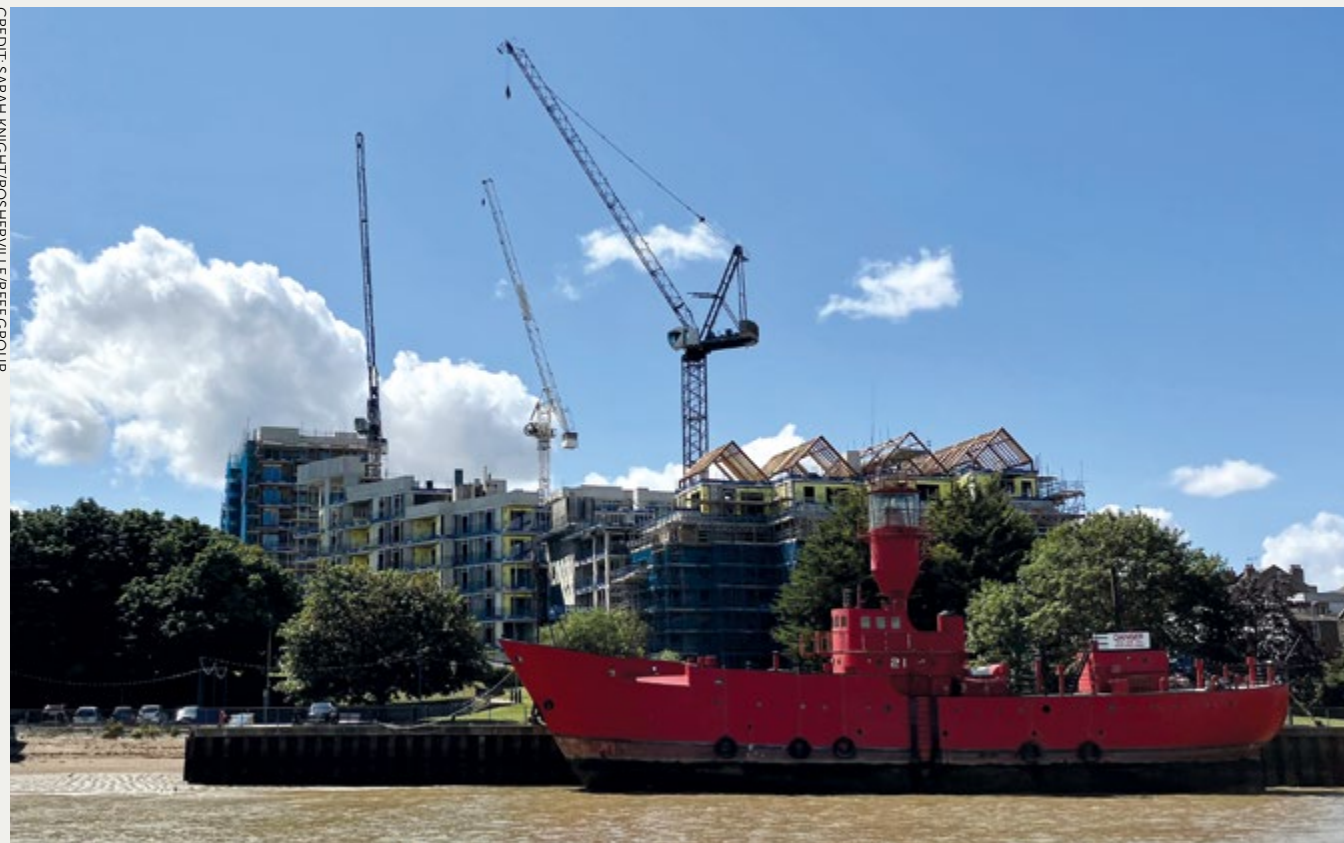
Under construction: The Charter development, Gravesham Riverside, Gravesend.
