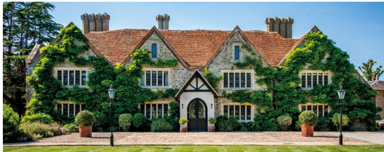
The restored 17th century house, Boys Hall, Ashford.
