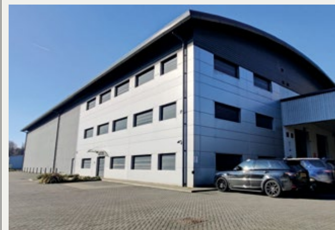
Hochiki Europe's new site at Apex House, Gillingham.
