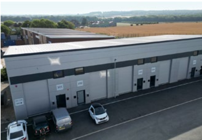
18 units (each 1,000ft 2 ) completed in September at Joseph Wilson Industrial Estate, Whitstable.
