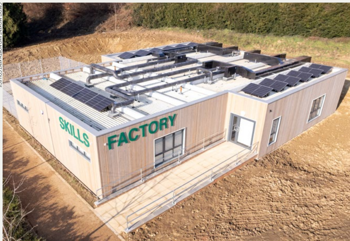
MidKent and North Kent College new 'Net Zero Skills Factory', Maidstone Campus.
