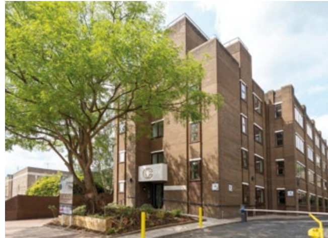
The substantially refurbished Crescent Court, Tunbridge Wells.
