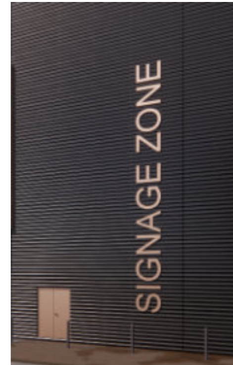
Signage Zone design with horizontal profiled panels
