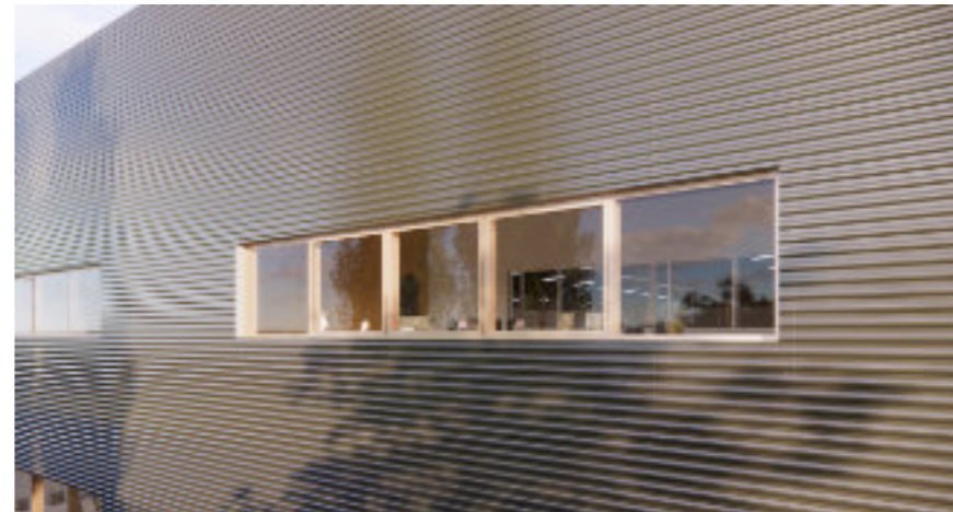
Glazing to North elevation
