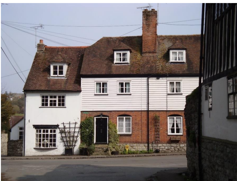
Figure 4 - Loose Valley Conservation Area
