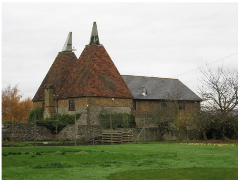
Figure 6 - East Farleigh Conservation Area
