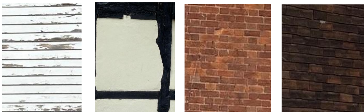
Fig 20: Notable materials in the area include timber, weatherboard cladding, brickwork and tile hung cladding.
