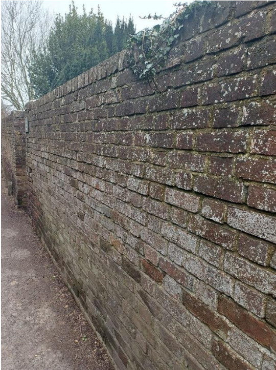
Figure 26 Brick wall in Lower Road
