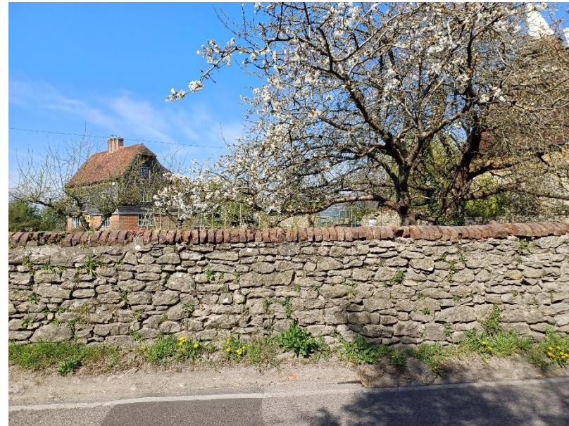
Figure 25 Ragstone wall in Dean Street
