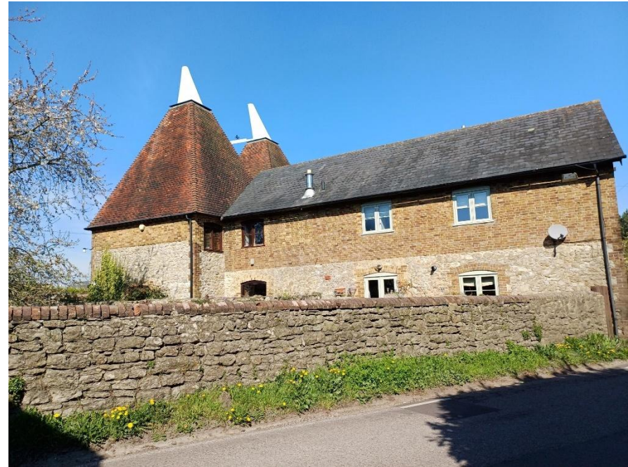
Figure 29 Kent peg tiles and slate tiles on the same building
