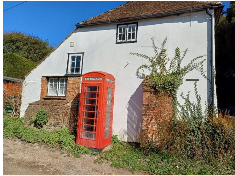
Figure 21 K6 Telephone Kiosk in Forge Lane
