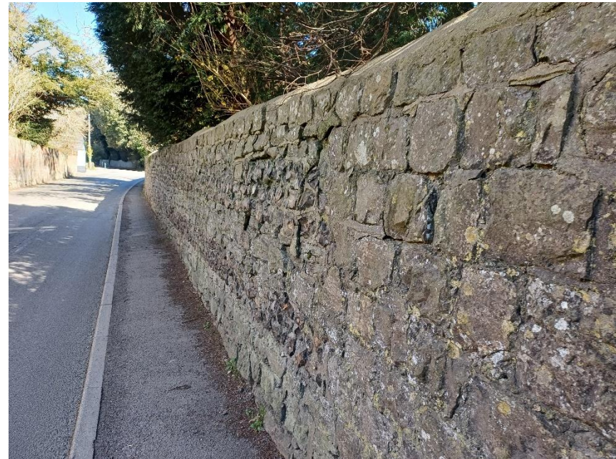
Figure 25 Ragstone Wall in The Street
