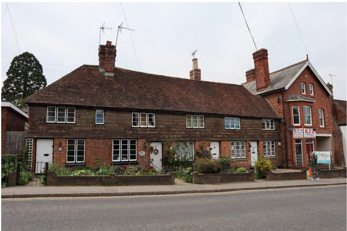
Figure 37 – Limes Terrace, with brick to the ground floor and hanging tiles to the first floor.
