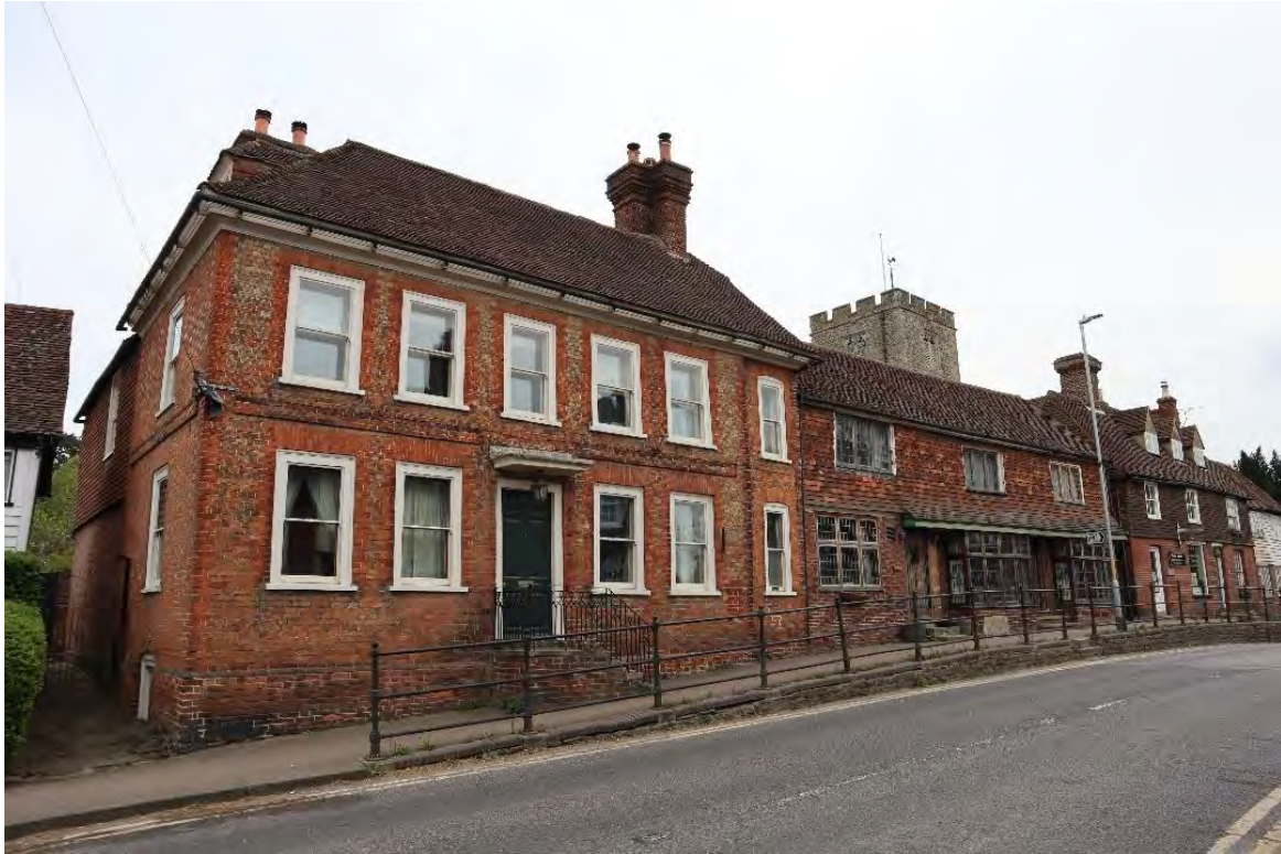
Figure 5 – The church tower peeps out from behind the terrace of mixed buildings (all Grade II listed). The architectural styles showing the development and wealth of the village.
