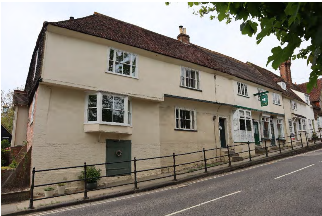
Figure 50 -painted render to timber framed properties.
