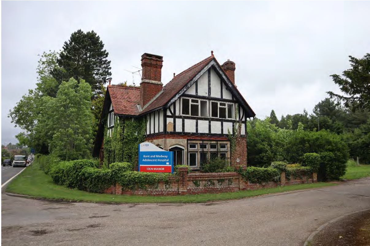
Figure 30 – Lodge to Iden Manor (at the time of the research was empty).
