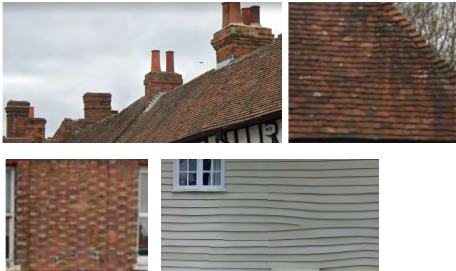
Figure 38 – examples of tiles, bricks, chimney stacks and weatherboarding.
