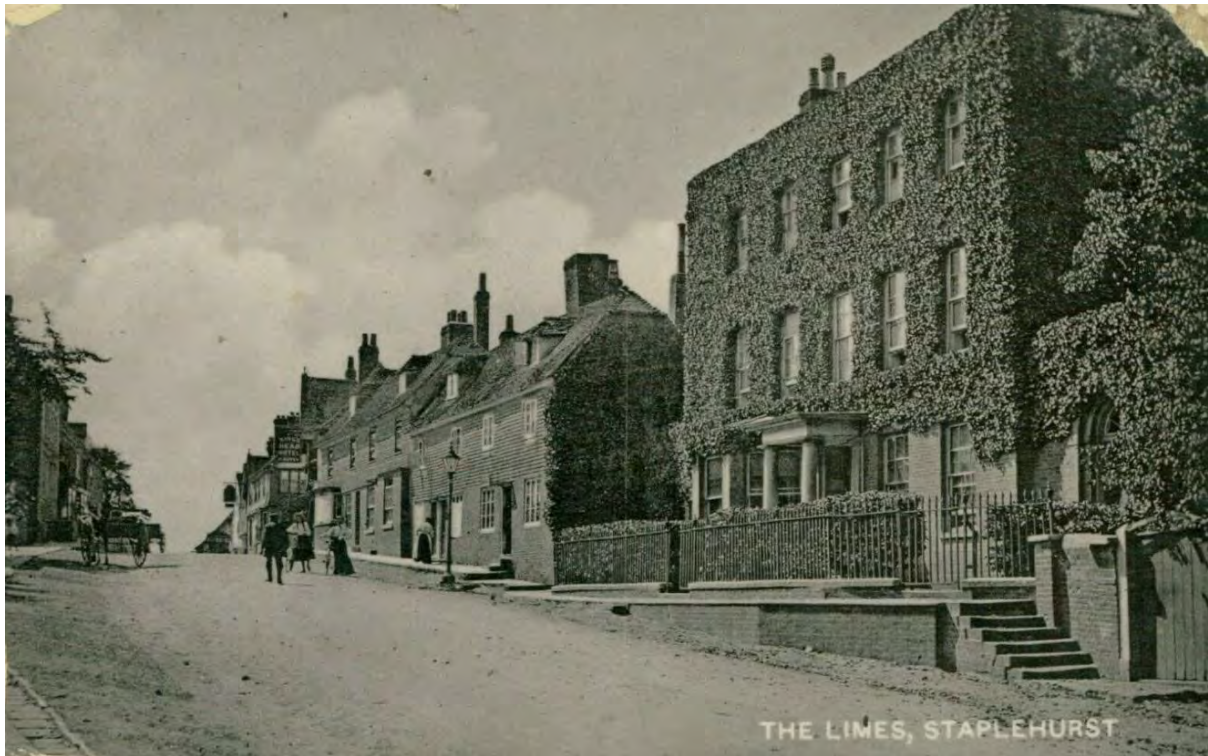
Figure 20 – Identified as The Limes on the image, but is Vine House, along High Street.
