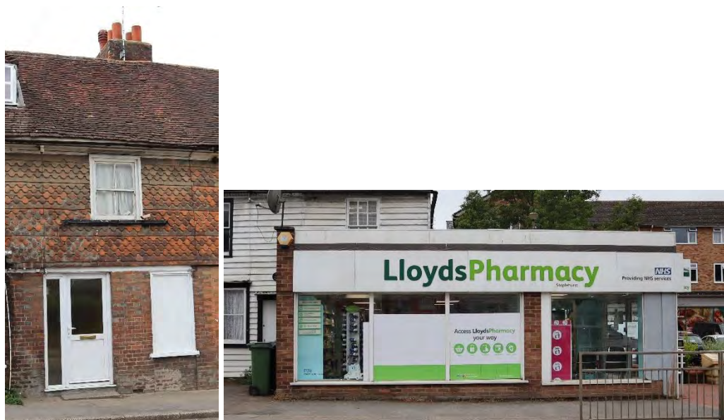
Figure 47 – UPVc door (now replaced) and blanked window to a traditional building and poor shop front which forms part of a listed building.
