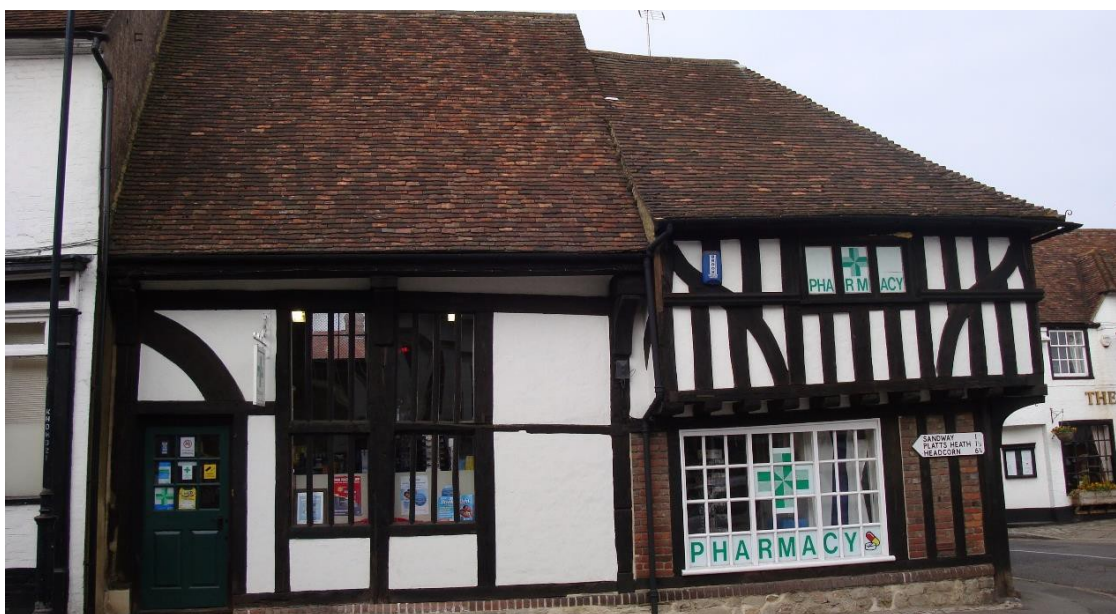
Part of a Wealden house survives in the High Street – the pharmacy in the High Street
