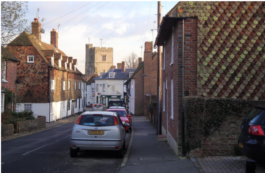
Maidstone Road showing a mix of materials – brick, render, Ragstone and tile hanging
