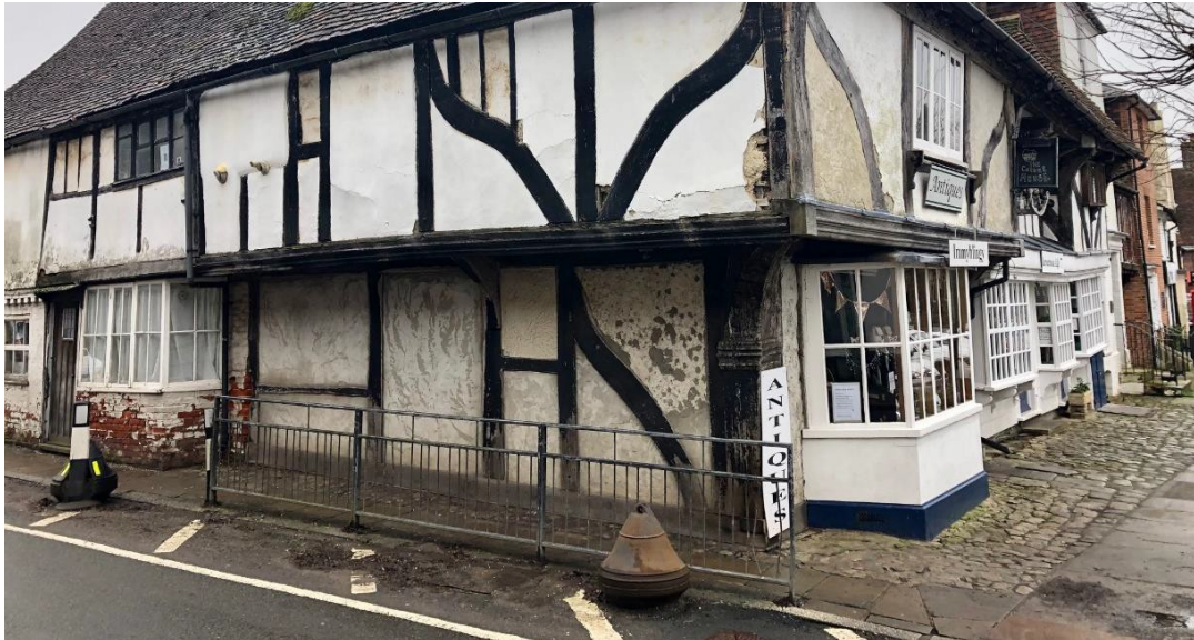
Poor quality railings and bollards on the north east corner of The Square
