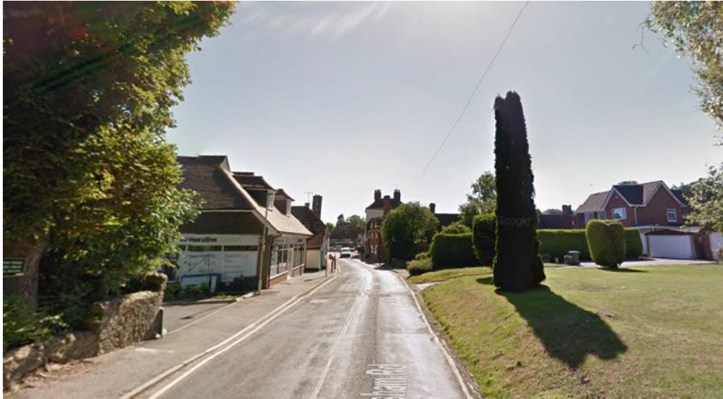
View looking towards The Square from Faversham Road
