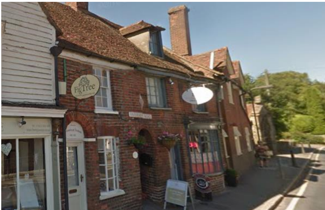
Satellite antenna and wiring on the front elevation within the conservation area
