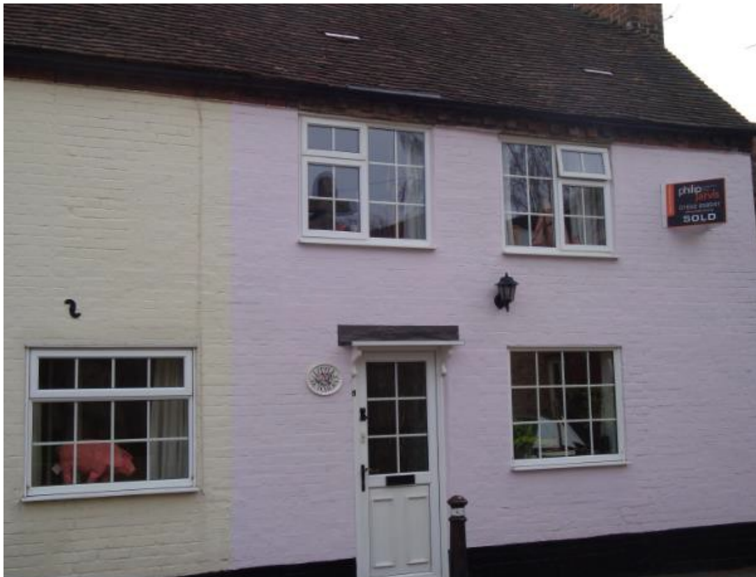
View of a property on the High Street showing Inappropriate replacement windows
